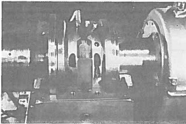
ASSEMBLED BEARING WITH CASING TOP REMOVED
