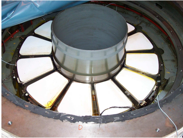
Fig. 13 Ffestiniog Unit 4 Thrust Bearing
